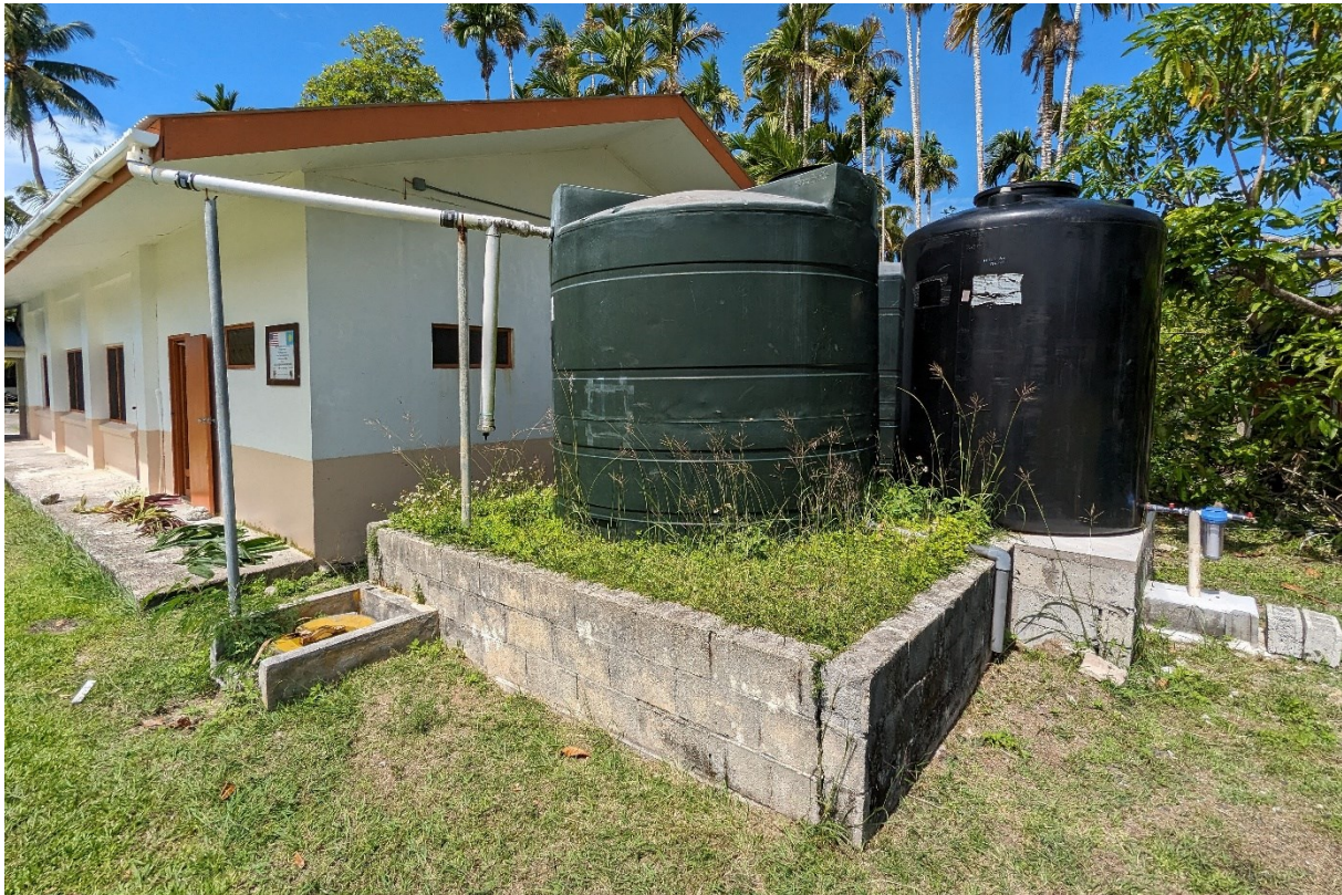
Figure 4: Original rainwater catchment system
